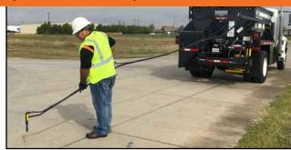
The Pivot Tack System helps operators stay safe by keeping hoses off the ground.
