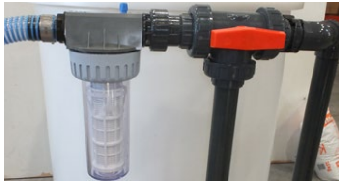
Heavy duty filter and 3-way valve
