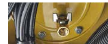
Fuel tank drain valve.
