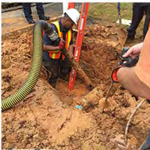
Power Vacs at work (Potholing)
